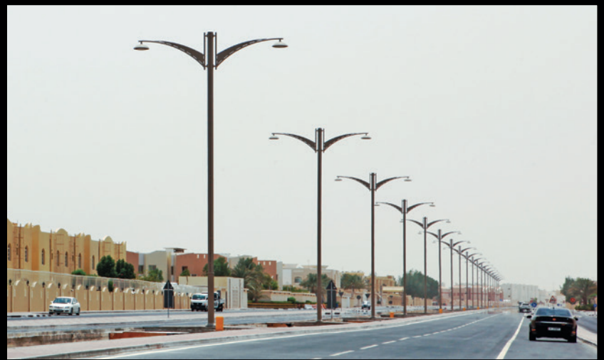
QATAR • AL WAAB CITY ROAD
